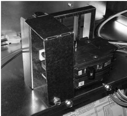
Figure 5. Line Cover Installed
