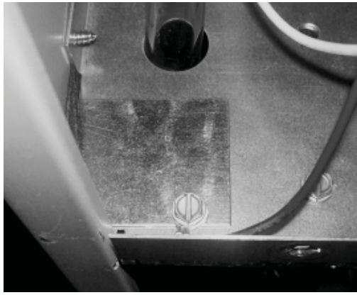
Figure 8. Opening in Front Left Floor Panel of furnace Burner compartment, Covered and Uncovered.
