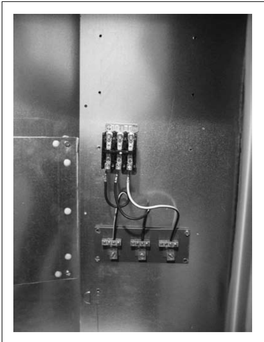
Figure 10. Single Contactor Mounting
