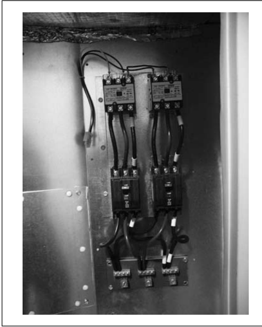
Figure 9. Circuit Breaker Mounting Plate Location
