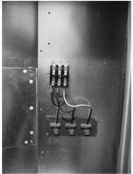
Figure 10. Single Contactor Mounting Location
